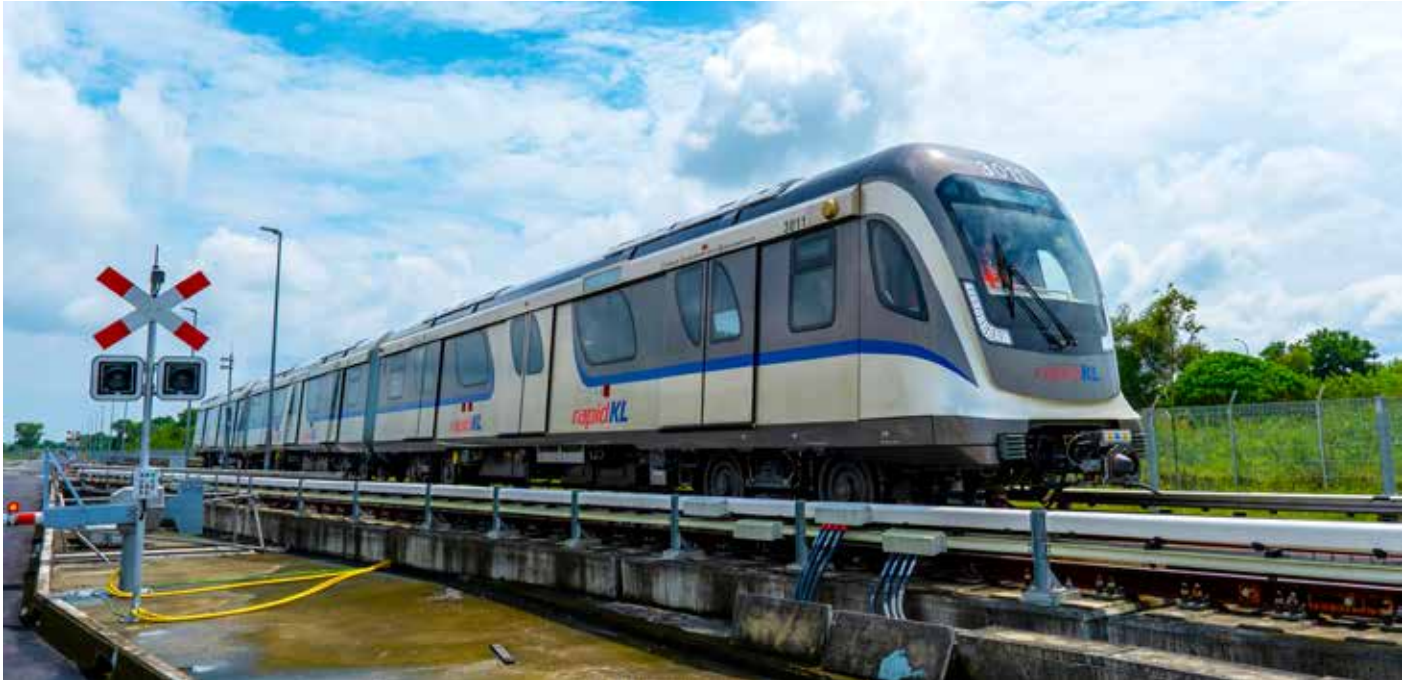
The Light Rail Transit 3 (LRT3) project, a significant infrastructure development project in our portfolio, achieved notable milestones in 2023. Almost all of the civil works were completed, achieving overall physical construction completion of 92% and financial progress of 88% at the end of 2023
