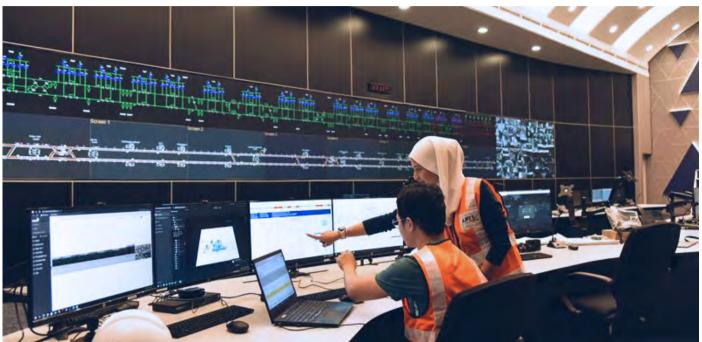
At the heart of the depot is the 34,091 sq. ft. Operation Control Centre (OCC). Inside is the Control Centre Room (CCR), which is vital for controlling, monitoring, and maintaining the trains once operations commence.
