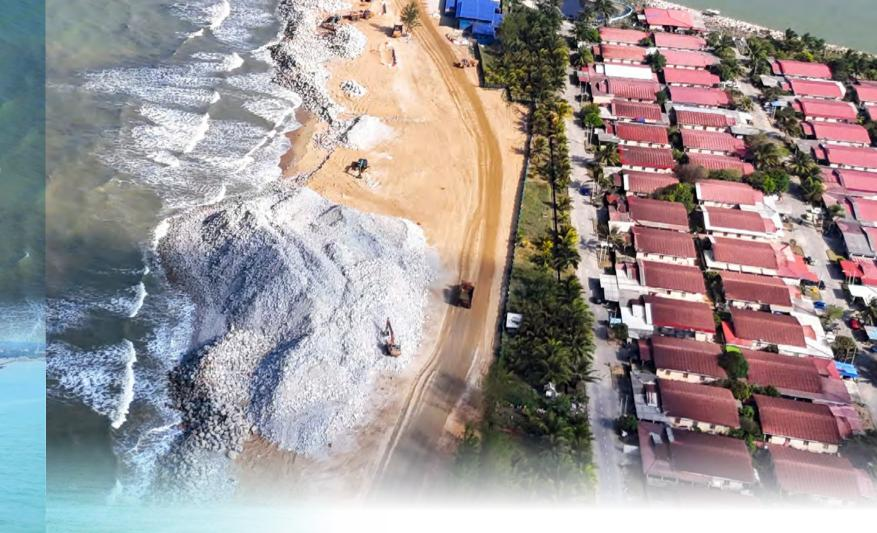
The project's specific scope includes the construction of 683.5 metres of the Northern Arm 1 breakwater and 682.55 metres of the Northern Arm 2 breakwater, along with four dykes, two beacon lights for maritime safety, and a navigational channel dug out to a depth of 2.5 metres below the low tide level (measured from Chart Datum, a standard reference point for water depths), promising safe passage for vessels and enhancing local economic prospects.
