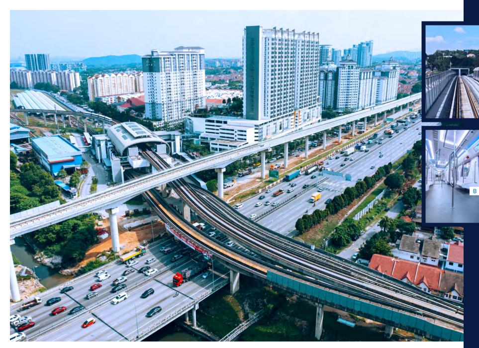
The project's long-span structures, a significant feature of the LRT Shah Alam Line, were strategically designed to optimise the alignment and minimise the number of piers required. The successful completion of 17 long-span structures, varying from 35m to 108m, are seamlessly integrated with U-trough girders employing advanced engineering techniques, ensuring the structural integrity and durability of these longspan structures.
